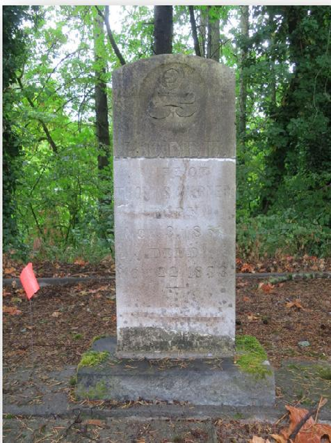
COMPLETED: Repaired three breaks with Akepox epoxy.
