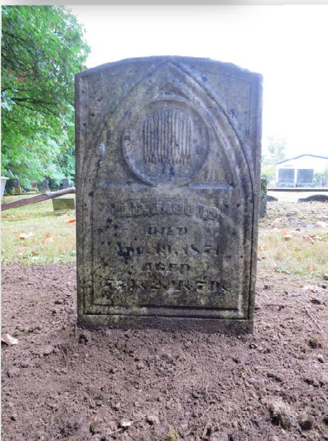
COMPLETED: Uncovered original slotted base in front of stone, determined stone bottom edge too uneven to reinsert in slot, stood stone upright at front of base on bed of 3/4" minus gravel, and packed in.
