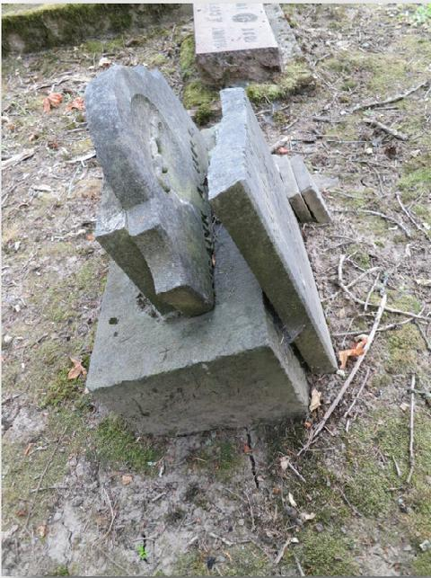
TO DO: Repair three breaks, two of which are old glue breaks.
