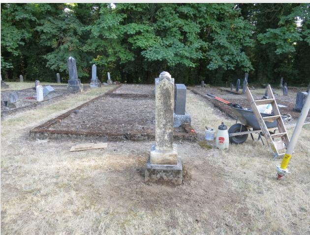
COMPLETED: Found marble footstone while leveling base and placed footstone next to base. Levelled on bed of 3/4" minus gravel, packed in, and reset stone in lime mortar.
