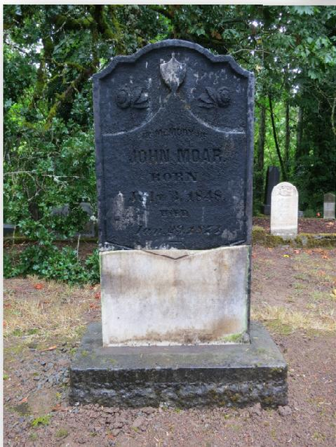
COMPLETED: Leveled on bed of 3/4" minus gravel, packed in, and repaired break with Akepox epoxy.
