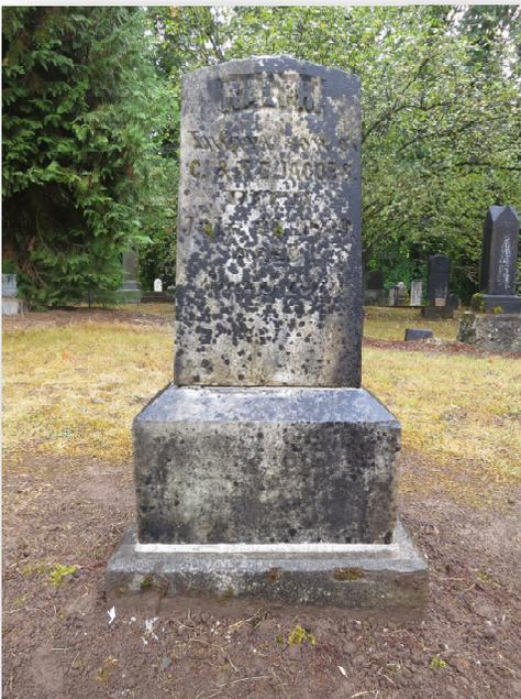
COMPLETED: Leveled base on bed of 3/4" minus gravel, reset plinth in lime mortar, and reset stone in Akepox epoxy.
