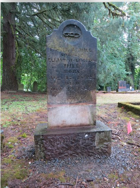
COMPLETED: Levelled base on bed of 3/4" minus gravel and repaired two breaks with Akepox epoxy.
