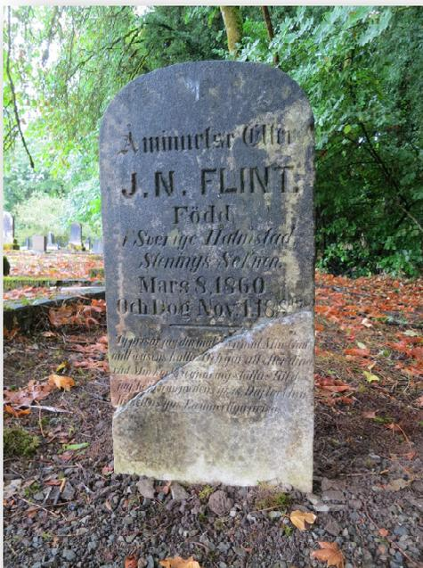
COMPLETED: Found marker bottom was embedded in concrete, so left concrete attached and leveled on bed of 3/4" minus gravel. Repaired break with Akepox epoxy.
