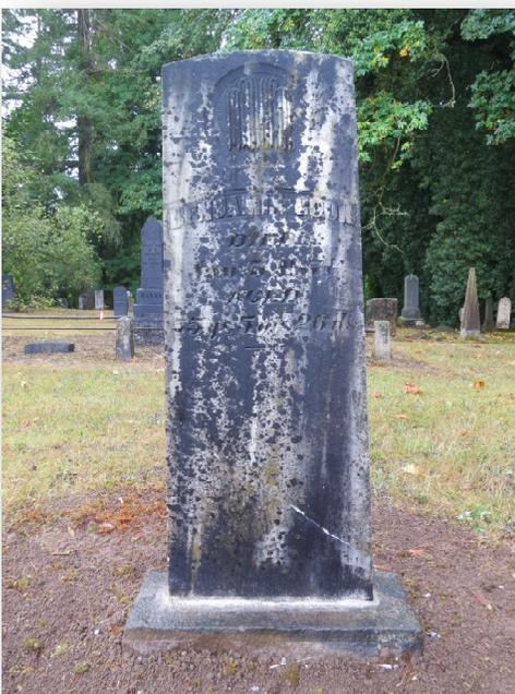
COMPLETED: Raised base 4" above grade, leveled on bed of 3/4" minus gravel, reset stone in lime mortar within base slot, and repaired break with Akepoxy epoxy.
