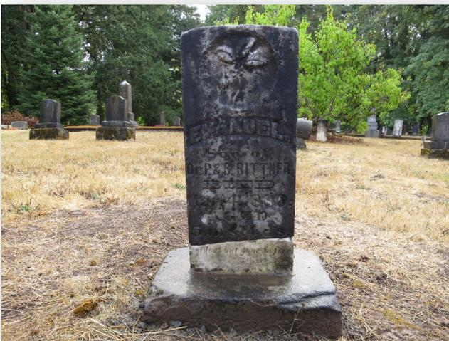
COMPLETED: Raised base 4" above grade, leveled on bed of 3/4" minus gravel, and repaired break with Akepox epoxy.
